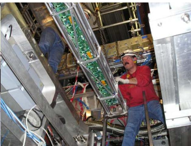
*A small part of the Tilecal drawers were refurbished on the surface outside the ATLAS cavern. The refurbishment process is shown on the right, while the drawer insertion in the Tilecal module, using the insertion tool produced at IFAE, is shown on the left*
