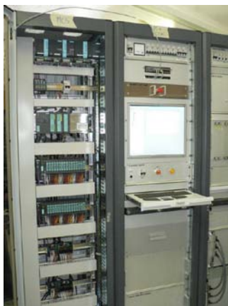
Figure 5 The magnet slow control system designed and built at the IFAE. The right rack holds the SIEMENS modules in charge of the monitoring.
