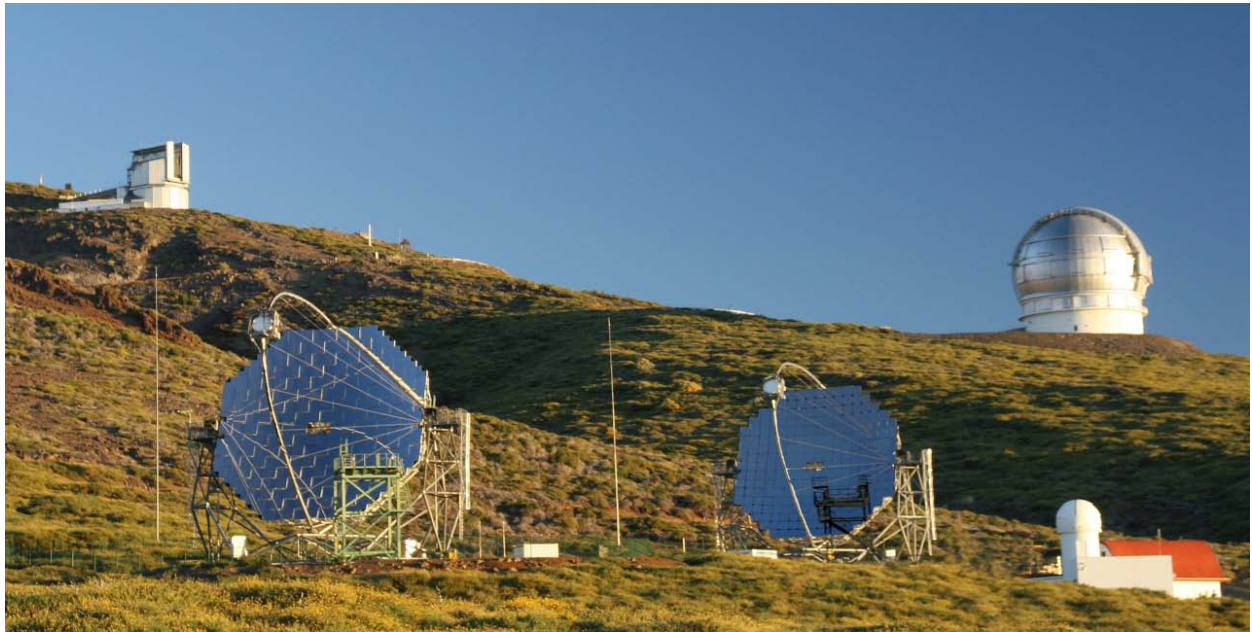
Figure 3 A picture of the two MAGIC telescopes after full installation of MAGIC-II (on the right) in Summer 2008 at the Roque de los Muchachos observatory. On the right, the electronics control building. The telescopes are currently in their commissioning phase and shall start regular operation in 2009. On the background, the domes of two optical telescopes: the Italian 3.6m Galileo Telescope (left) and the Spanish GRANTECAN 10.4m telescope (right).
